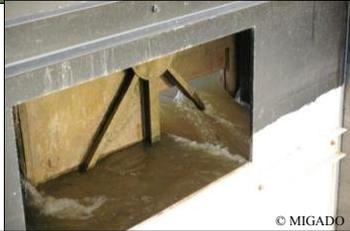
Telescopic gate allowing to keep a defined upstream water level
