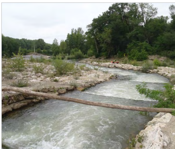
Figure 22 – Barrage de Barcelonne-du-Gers (MIGRADOUR)
